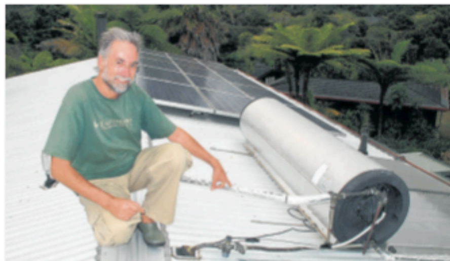
TOP TIPS: Rolf Mueller-Glodde with the resort's solar water heater (foreground) and photovoltaic solar panels, at rear. PICTURE / PETER DE GRAAF
